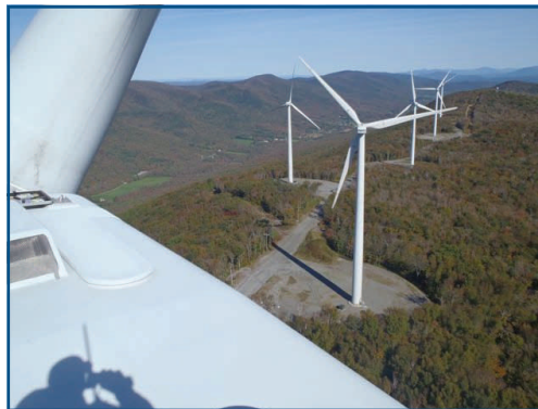
The shadow of MMWEC's Neil Geary can be seen at lower left atop a Berkshire Wind Power Project turbine. MMWEC performs a variety of maintenance and operations tasks at the project.
