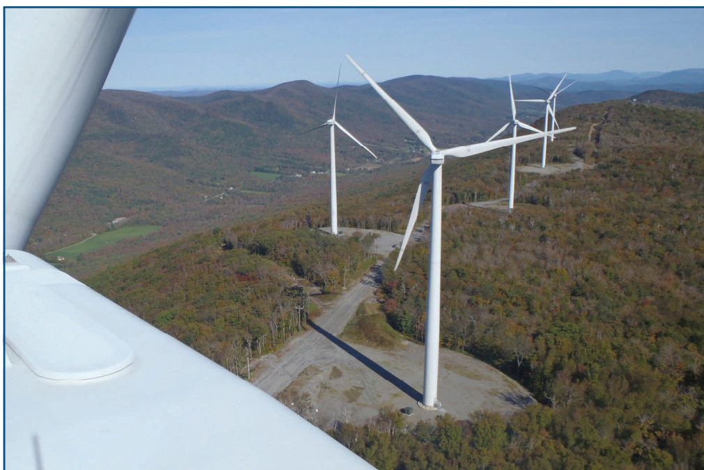
The above photo of the Berkshire Wind Power Project is featured in the American Wind Energy Association 2012 calendar for the month of January. About 12,000 copies of the calendar are distributed to 2,400 AWEA members, 300 media contacts, all members of Congress, regulators and other national audiences. More about Berkshire Wind on Page 3.
