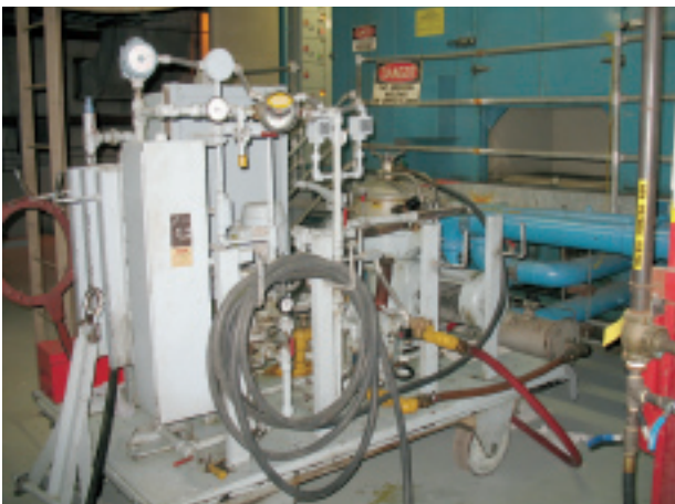
9. Varnish issues have surfaced only once in the plant's lifetime. Centrifuge cleans oil on each unit for one week in six
